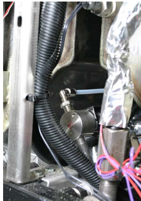
Figure 2: The solenoid, visible from the rear of the fryer (see arrow), must be rotated to the left to accommodate placement of the oil disposal activation arm.
