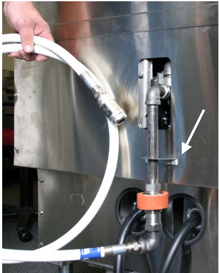
Figure 10: The oil discharge assembly is shown completely installed. The arrow marks the bracket used to secure the downspout.
